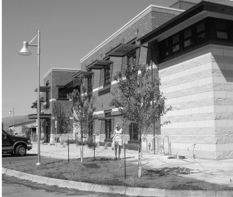
Figure 57 – Provide belt courses and horizontal trim bands of contrasting color to reflect each floor level. This technique will assist in creating a more human scale.
