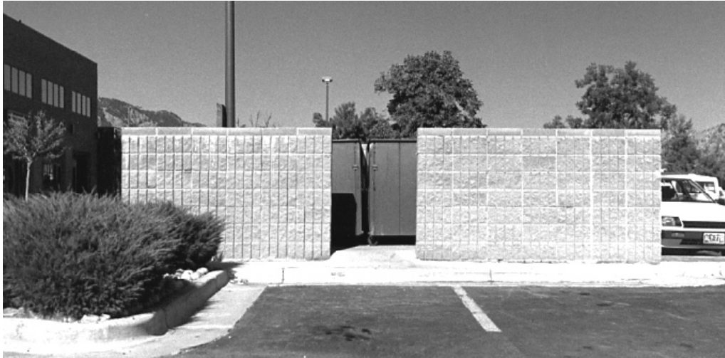
Figure 40 – Orient the door to a trash enclosure to face away from the street when feasible.
