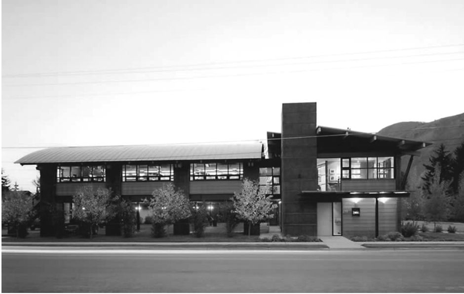
Figure 81 – Two story office.
