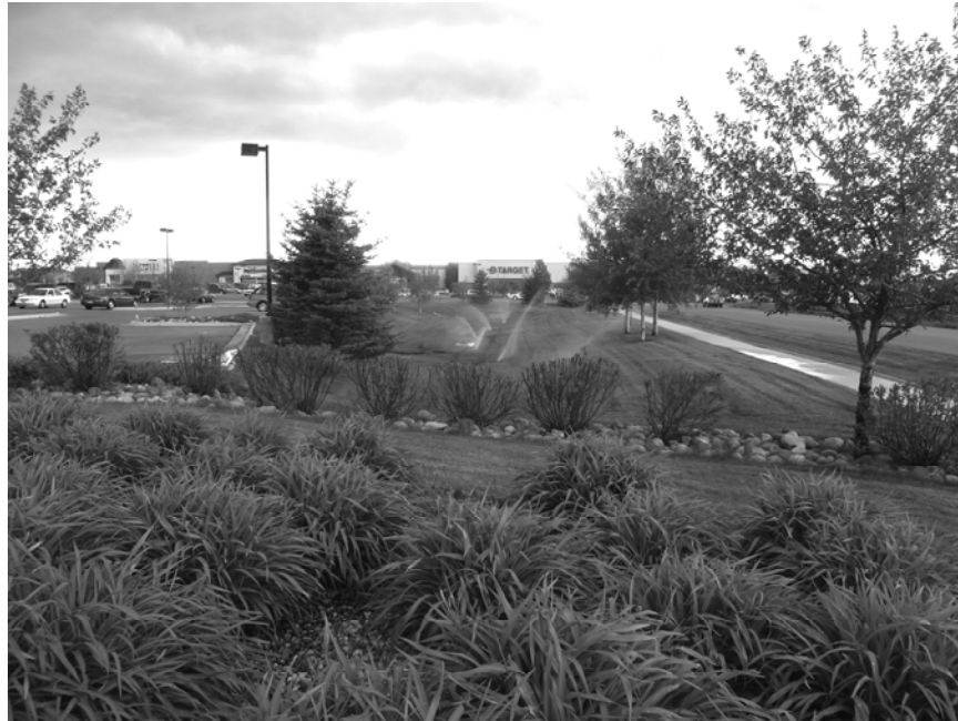
Figure 26 – Combining stormwater swales with landscape buffers along property lines creates an attractive green space.
