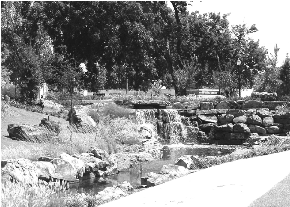
Figure 7 – Incorporate drainage and detention basins as site amenities and landscape design features.
