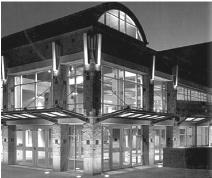
Figure 82 – Two story office.
