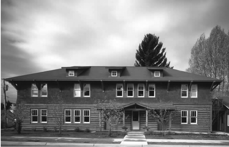
Figure 99 – Two story office building.
