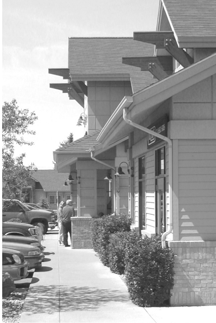
Figure 58 – Providing a variety of ridge line heights can assist in reducing the perceived scale of a building and is encouraged.
