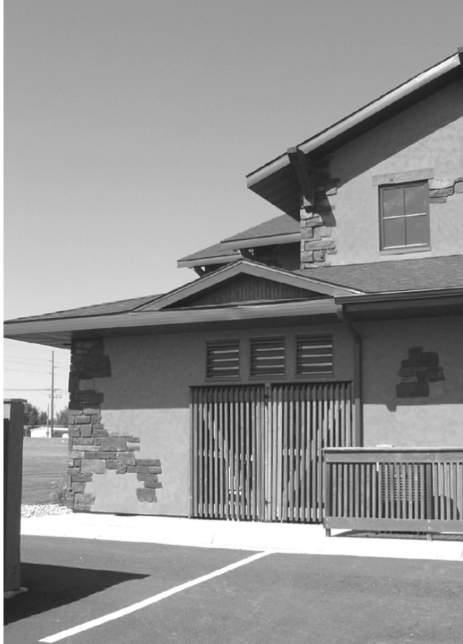
Figure 41 – Service area screens should be in character with the building and site.
