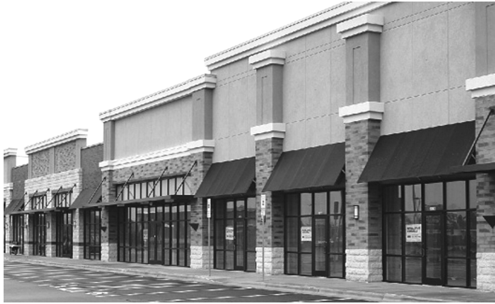
Figure 62 – Stucco-type materials may be appropriate if earth tone colors are utilized in conjunction with masonry accents.
