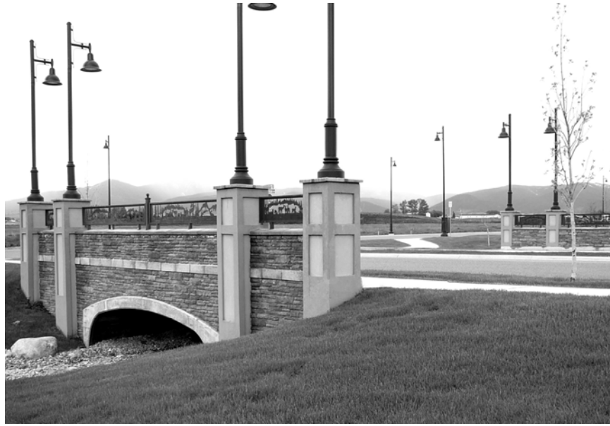
Figure 27 – Include site amenities to add interest to larger parking areas.
