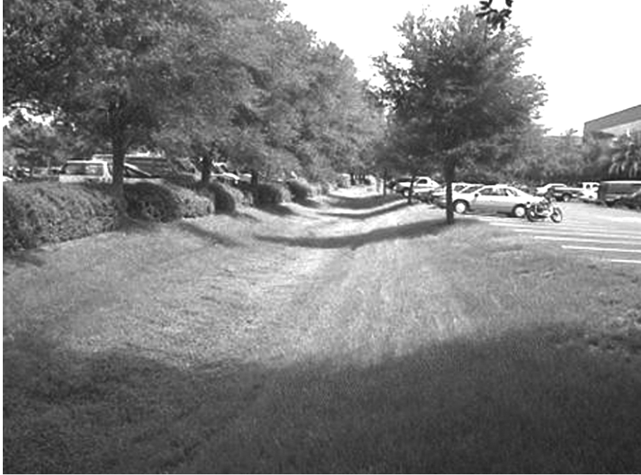
Figure 6 – Open storm water swales, such as the one above, are an excellent way of recharging storm water back into the ground.
