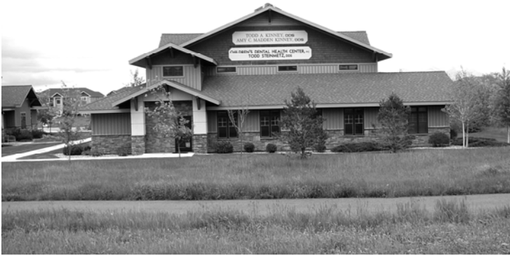
Figure 80 – Two story office.
