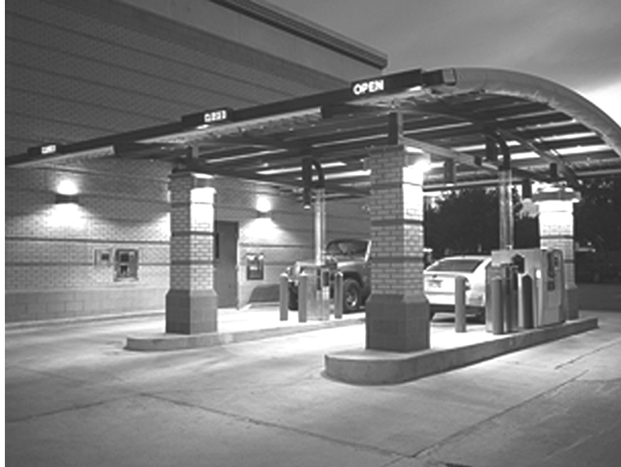
Figure 63 – Canopies that are independent of the main architectural structure should be low profile.
