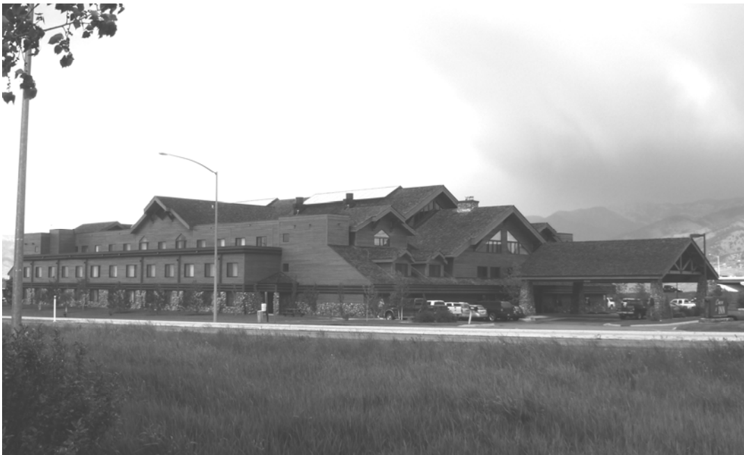
Figure 89 – Hotel with covered arrival court.
