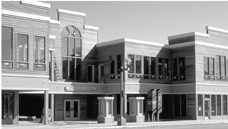
Figure 56 – Varied building forms assist in breaking up building massing and assist in providing a sense of human scale.
