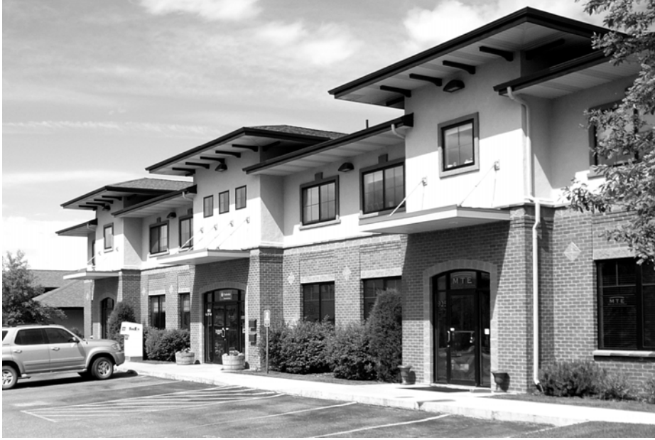
Figure 83 – Two story offices.
