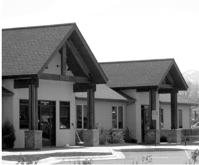
Figure 59 – Utilizing sloping roof forms can assist in reducing the perceived scale of a building.
