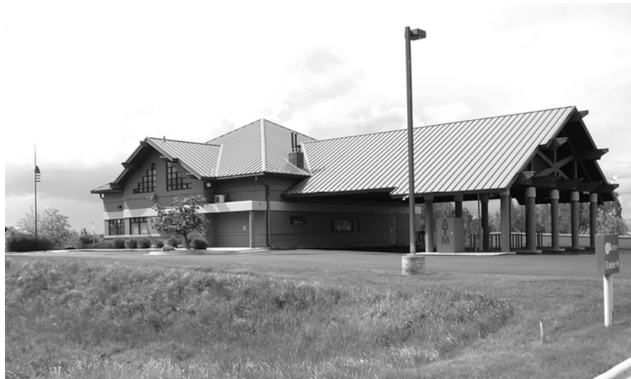
Figure 64 – Canopies that are part of the main building architecture should utilize the same roof forms and materials.
