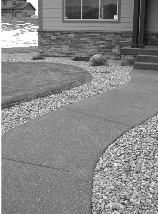
Figure 14 – Typical Curved Sidewalk of Exposed Aggregate.
