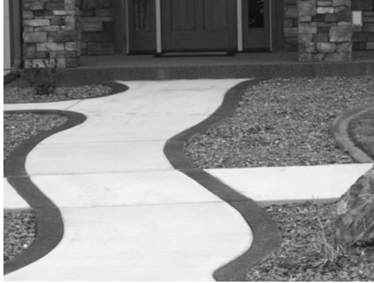
Figure 12 – Typical curved entry sidewalk with 6" color trim.
