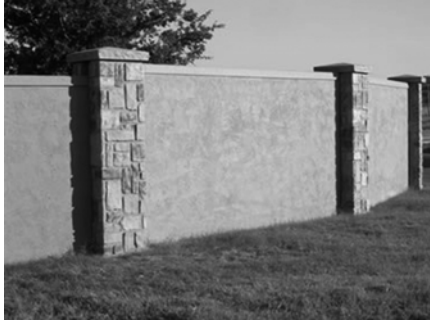
Figure 26 - Stucco-Type Wall with Stone Piers.
