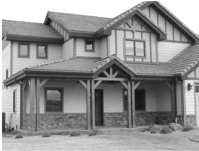
Figure 7 – Typical Trim Board and Beams.
