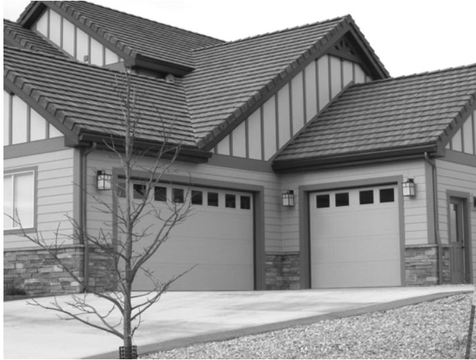
Figure 9 – Third Garage Bay Offset from Main Garage.
