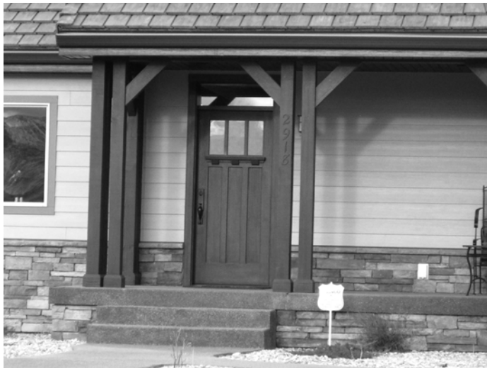
Figure 15 – Stone Porch with Decorative Concrete.
