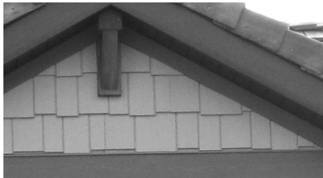
Figure 6 – Craftsman Exposed Brace on End Gable.
