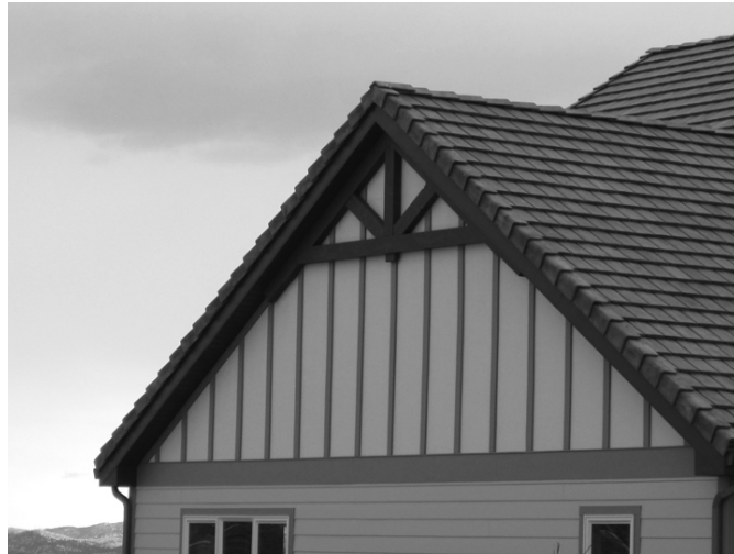
Figure 5 – Craftsman Exposed Structure Detail on End Gable.
