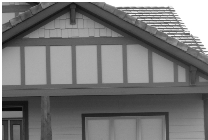
Figure 8 – Typical Trim Board Details.
