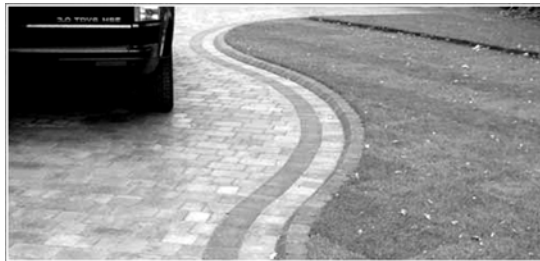
Figure 13- Typical Curved Driveway of Modular Pavers.
