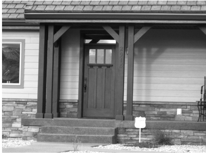
Figure 3 – Craftsman Posts and Braces on Porch.
