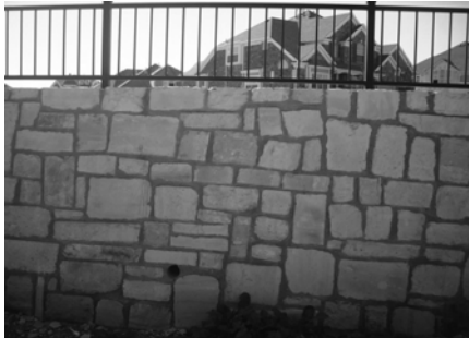
Figure 28 – Stone Wall with Metal Railing.
