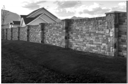
Figure 27 – Stone Wall with Stone Columns.
