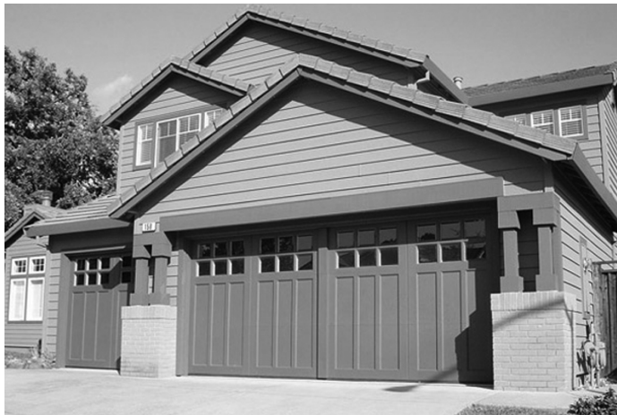
Figure 10 – Third Garage Bay in an Offset Wall Plane.
