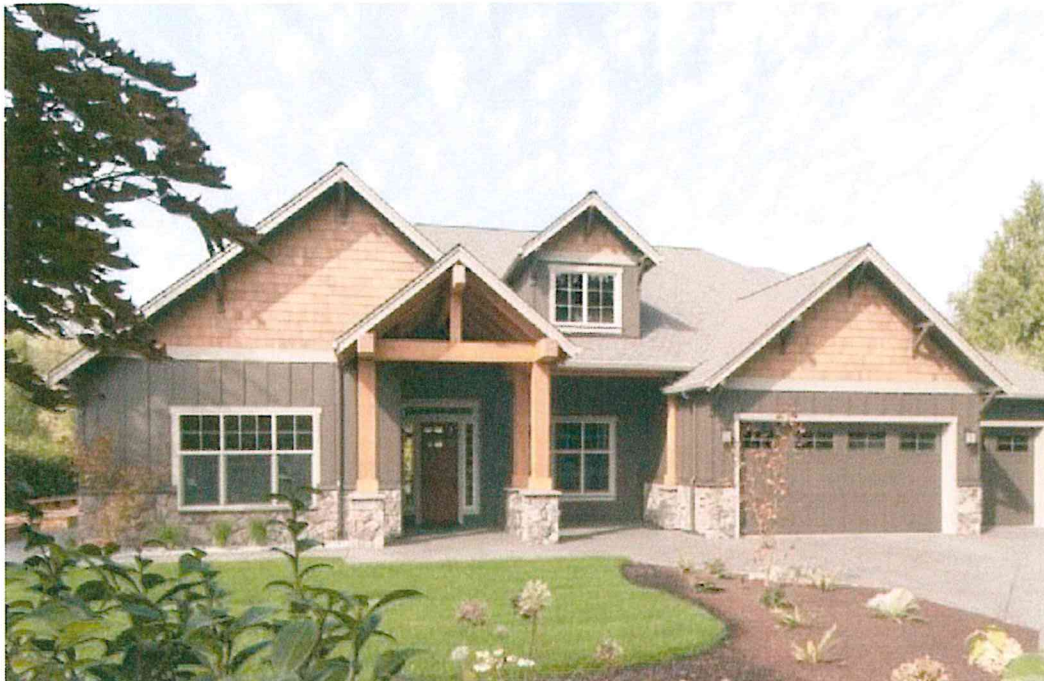
Craftsman with Hipped Main Roof and 3-Bay Garage
