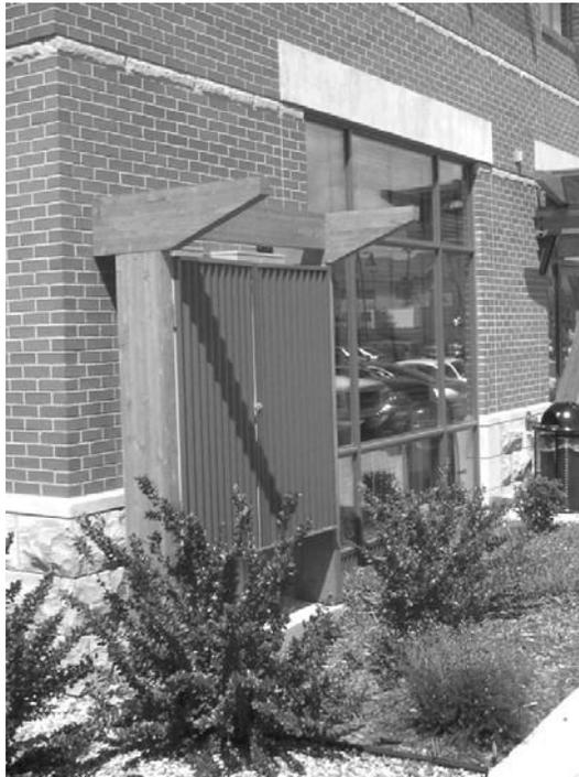
**Figure 65 – It is appropriate to integrate equipment panels into the building design.**
